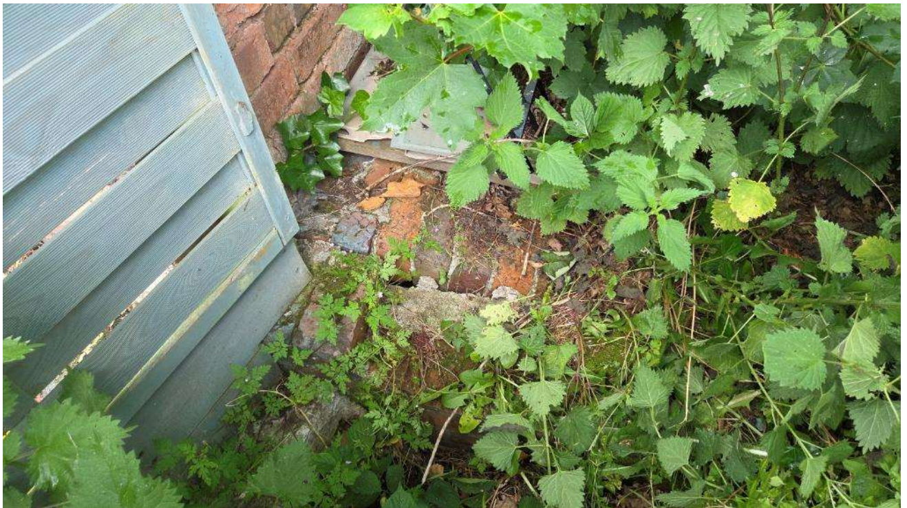
13) Potential brick counterfort to rear of the store at the end of the fence, (churchyard side).
