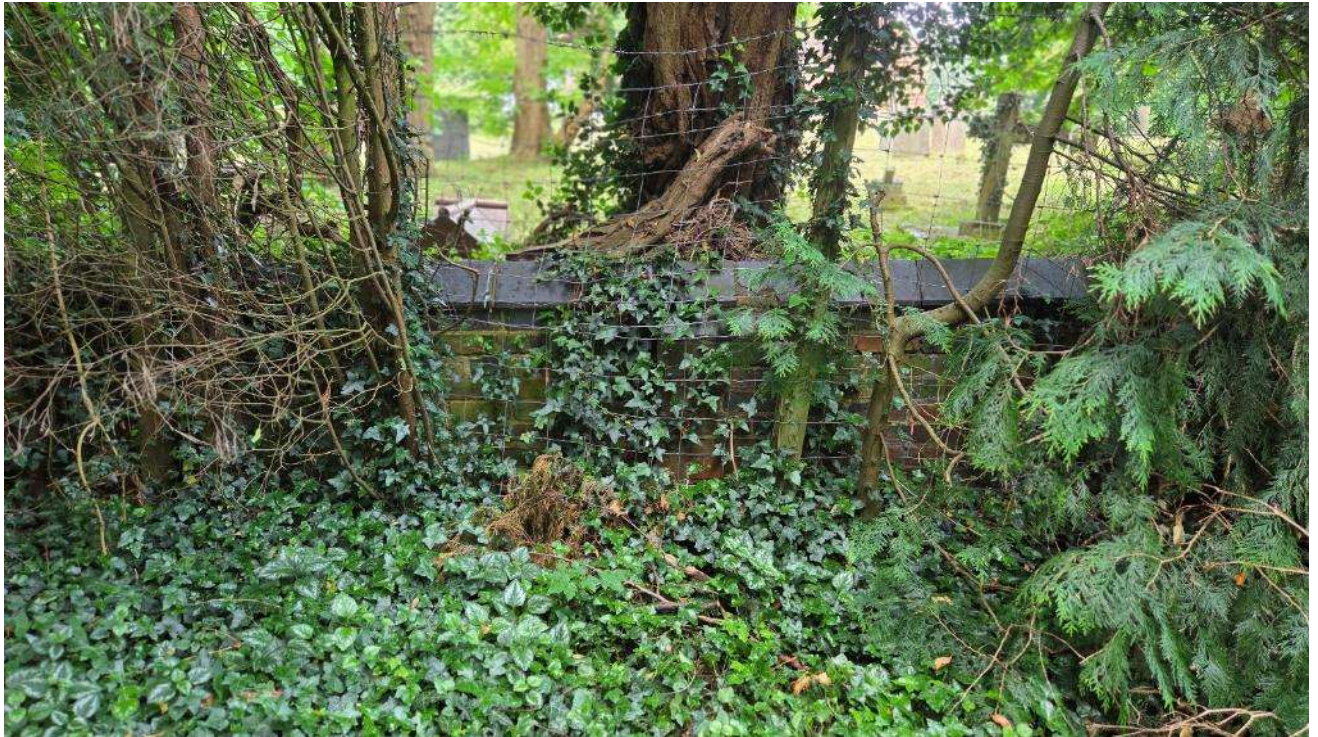
24) Low retaining wall section to east boundary.
