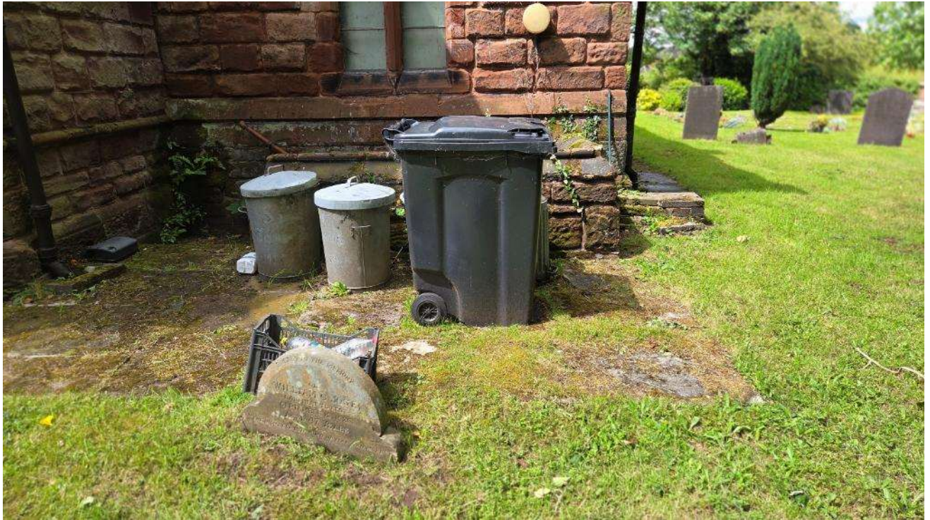
40) Below ground store accessed from staircase by church.
