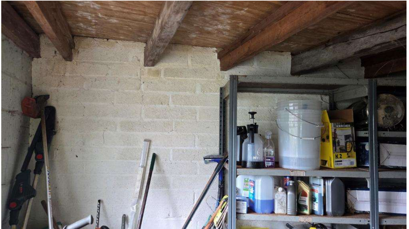
10) Eastern section of outbuilding; retaining wall obscured by new block wall built in front.
