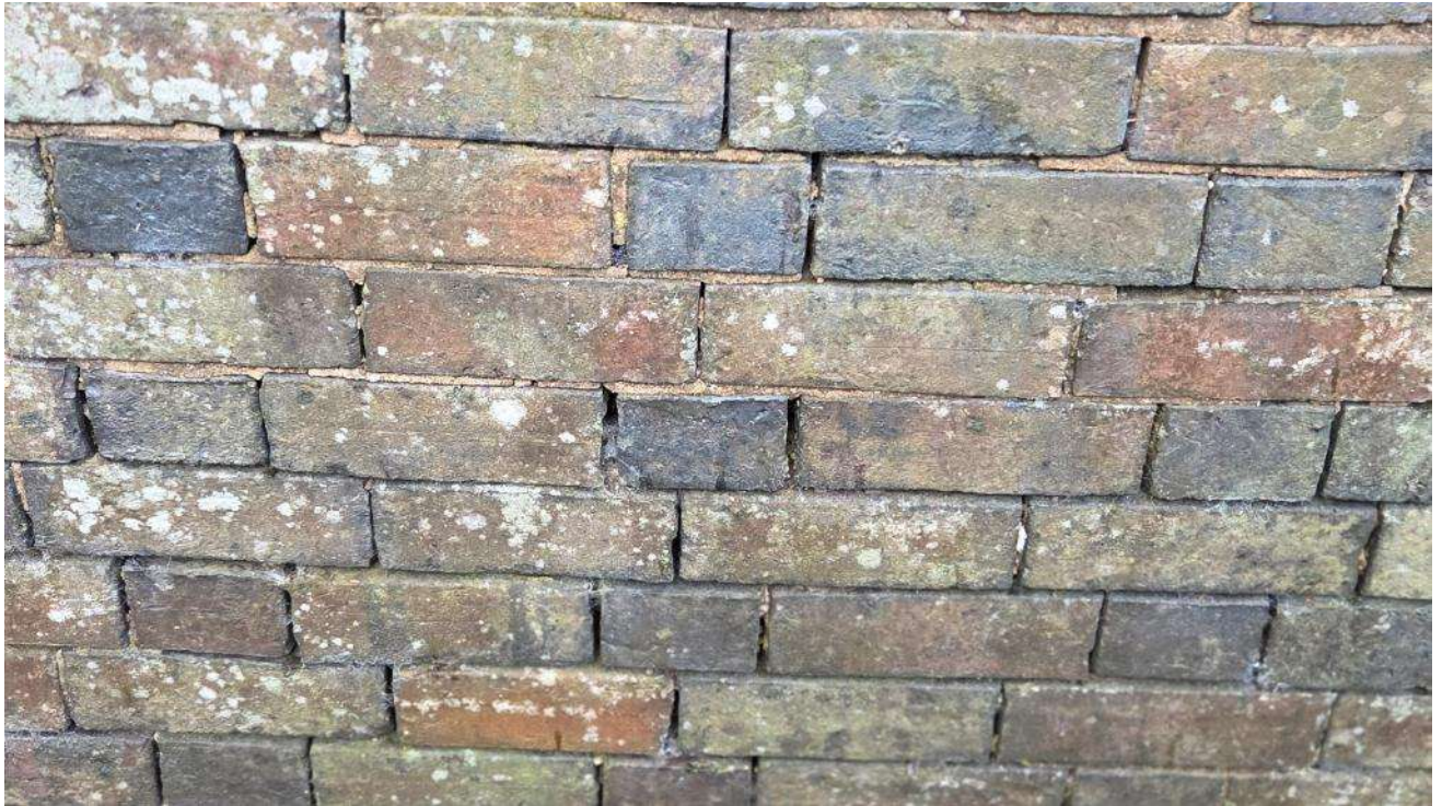
34) Typical open jointed section of wall to central and southern end.
