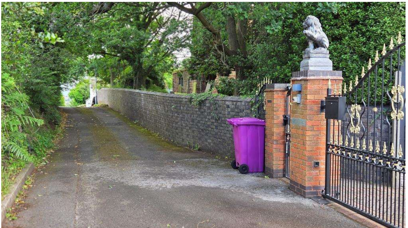
37) View looking north back to lamppost. Retaining wall seen curving behind gates of the property and the first concrete post of a timber fence to the far right.
