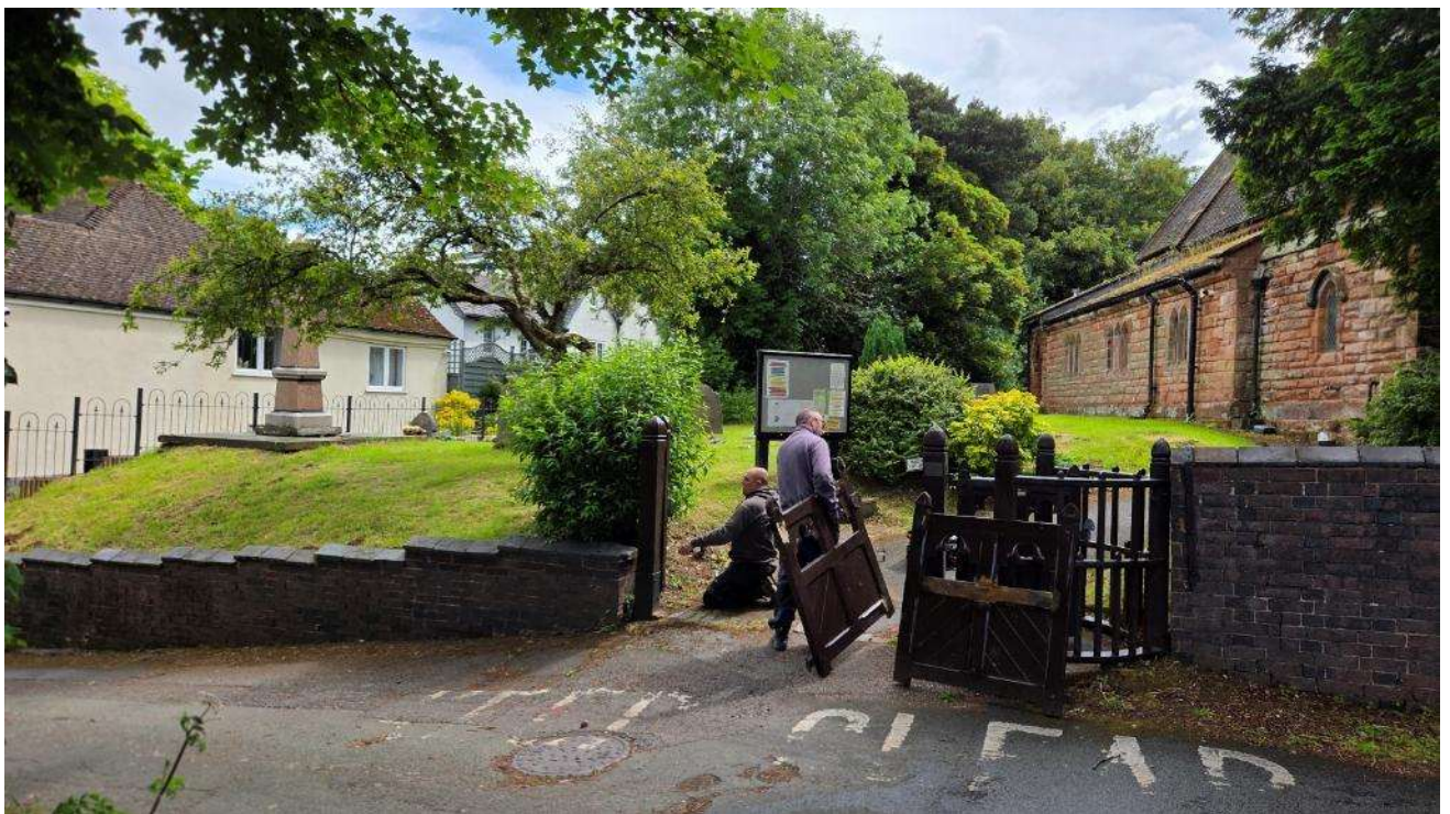
27) Gates being refurbished.
