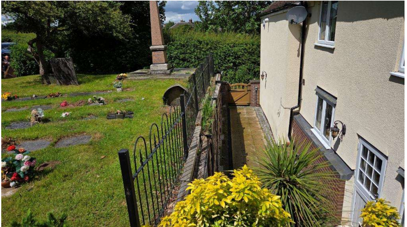
3) View looking west with graves close to retaining wall.
