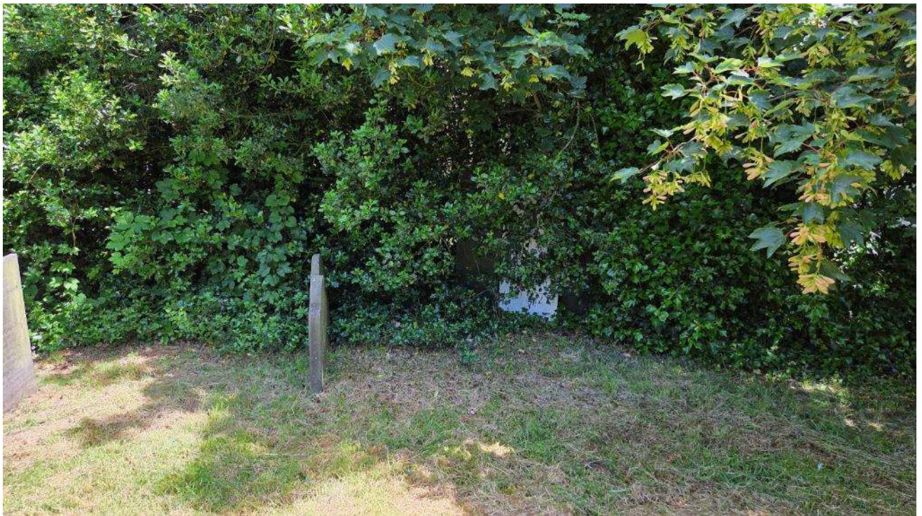
39) Overgrown vegetation innaccessible boundary facing north to the Old Rectory
