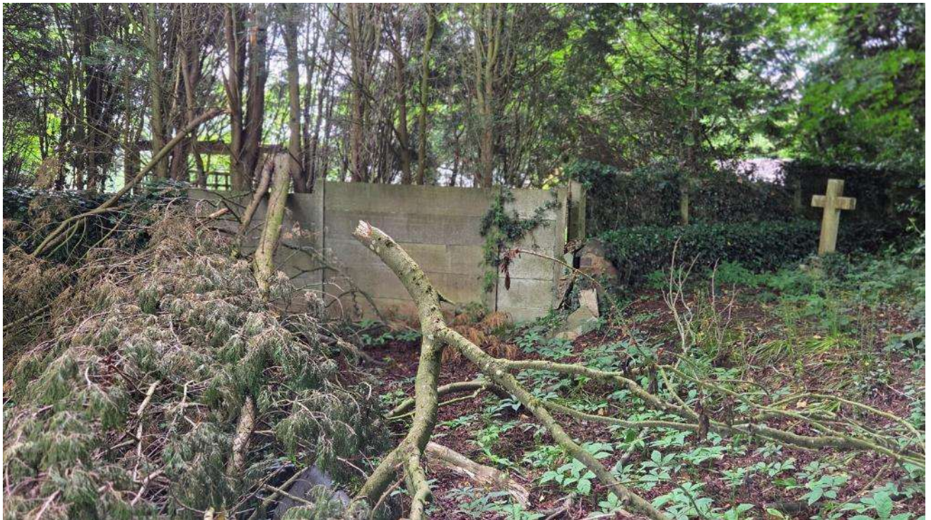
47) End of the south brick boundary wall with new precast wall section to the left (further east).
